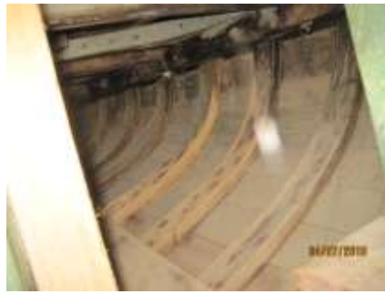
Framing in Port Quarter
